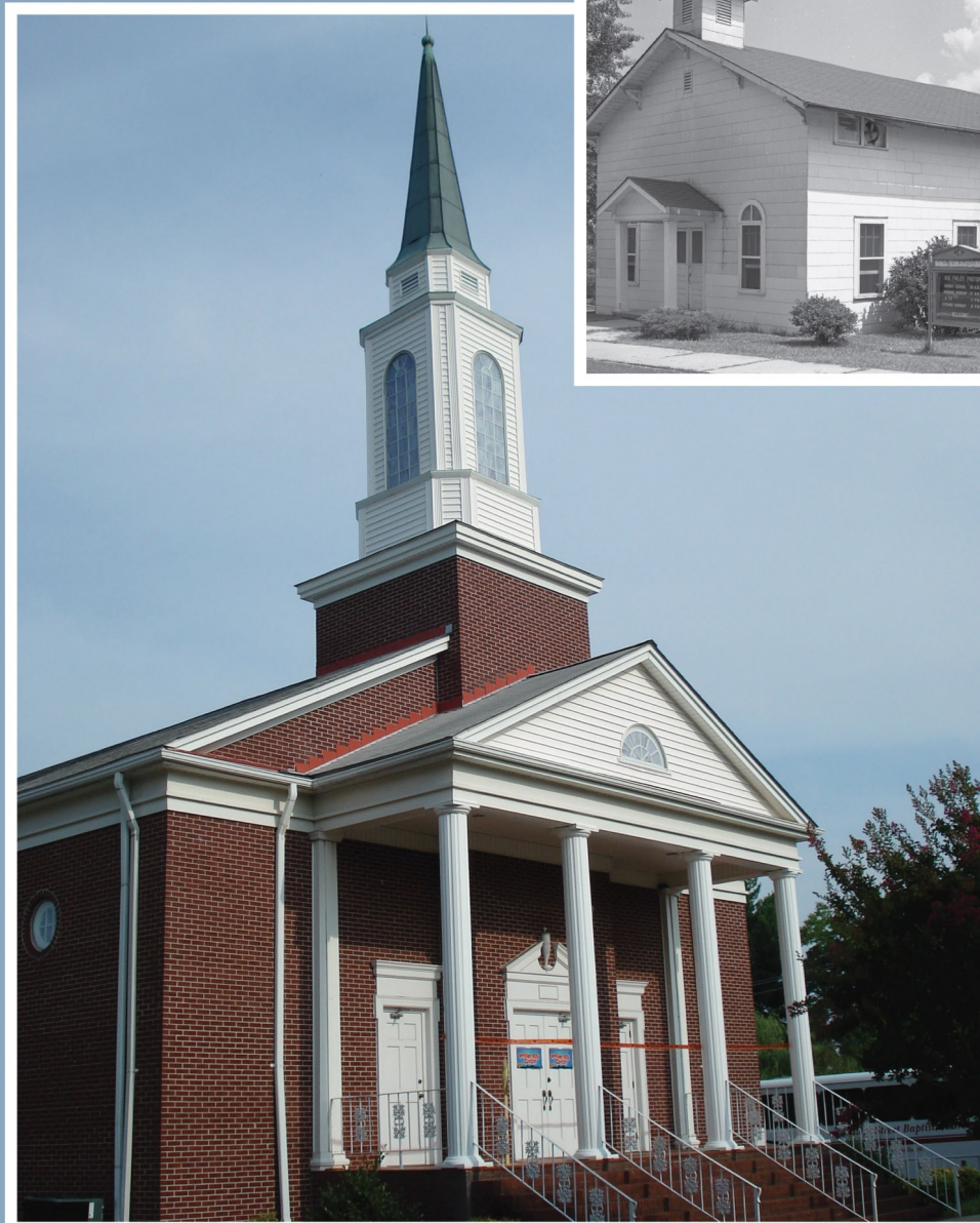
College Street Baptist Church Walhalla, South Carolina November 8, 2009
